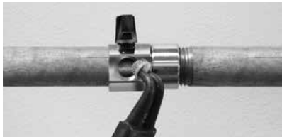
Remove the filter with pliers then clean or replace it
